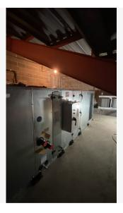
New air handler setting in place. The new units are larger than the old.
