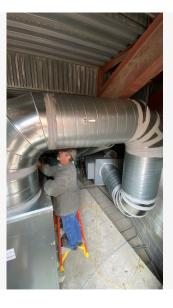
New ductwork installed. Maintenance no longer has to climb over the ductwork!
