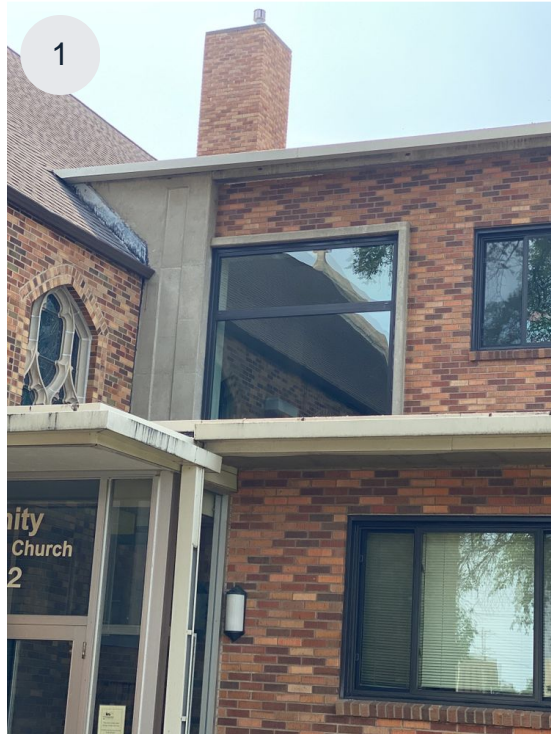
New high efficiency window above the stairwell.
