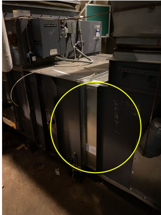
New cooling coil is installed.
